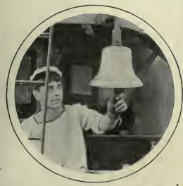
THE NEW BELL OF THE "BROKE." Cast from the lid of a Torpedo Tube of G42.
